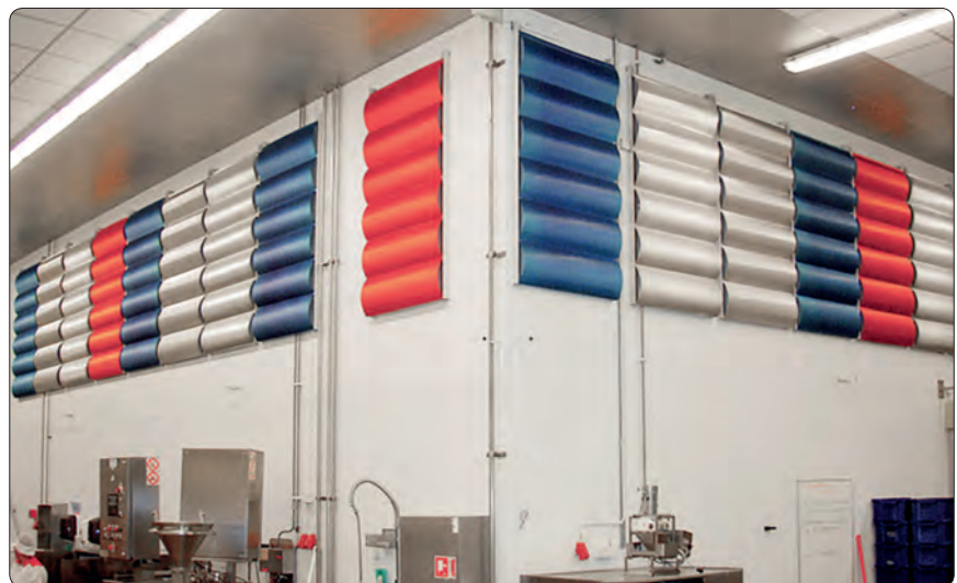
The post formed "Noise Resist" absorbers are attached to hinged wall frames so that they can be steam cleaned from both sides.
