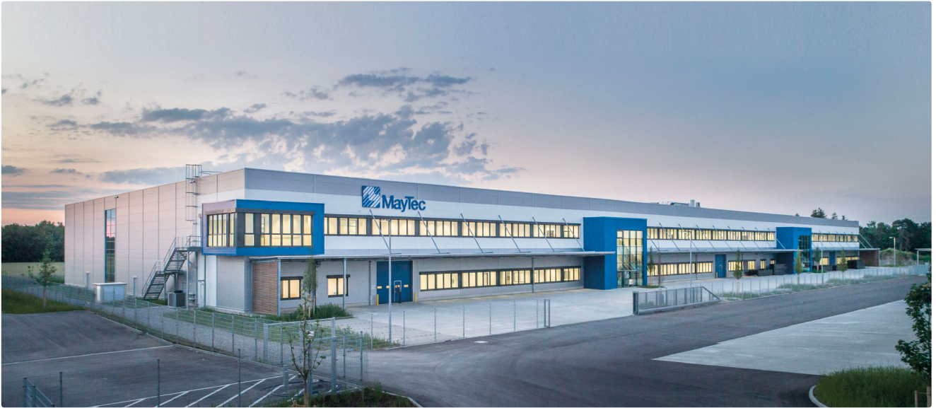
MayTec GmbH plant in Olching
